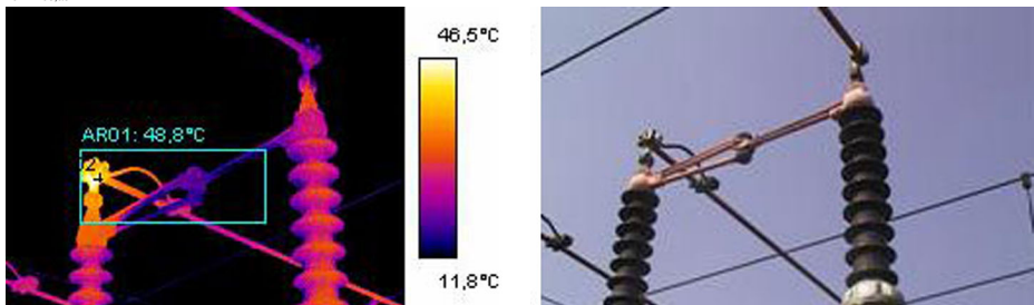
Figure 28.1 An infrared and a visual image of a power line isolator
