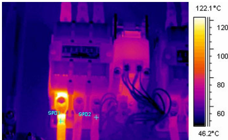
Figure 28.9 An infrared image of indoor electrical equipment (2).
