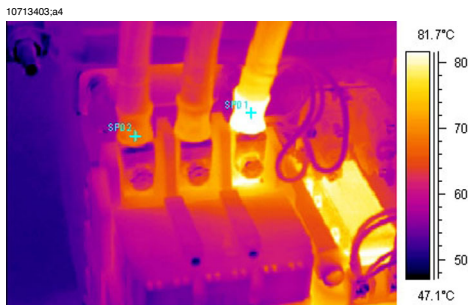
Figure 25.8 An infrared image of indoor electrical equipment (1).
