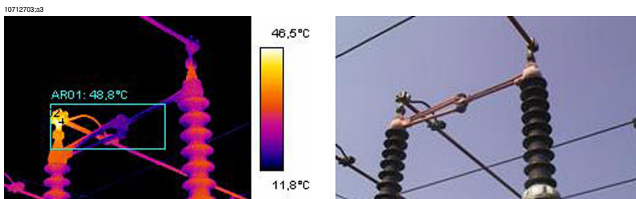
Figure 31.1 An infrared and a visual image of a power line isolator
