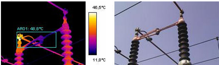
Figure 17.1 An infrared and a visual image of a power line isolator
